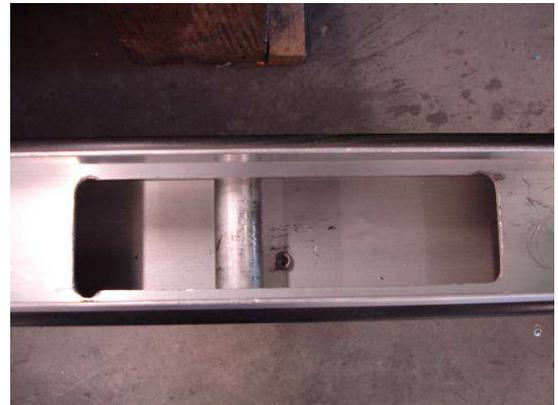
Fig. 03 (Anchor bolt on stop log)
